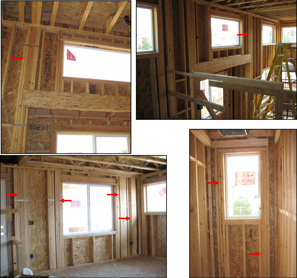
Figure 10: Examples of side-by-side stud bundles
